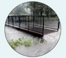
FOOTBRIDGE BY THE RIVER SILNICA
