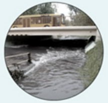
PASSAGE UNDER BRIDGE
